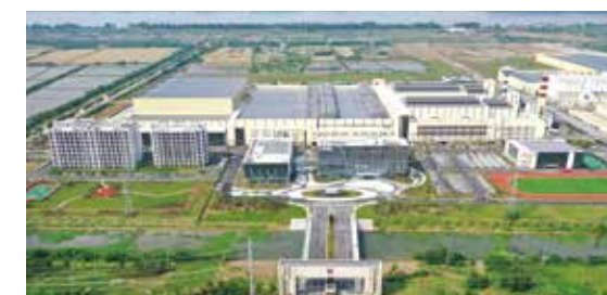
Newly completed Jiujiang Intelligent Production Base.
