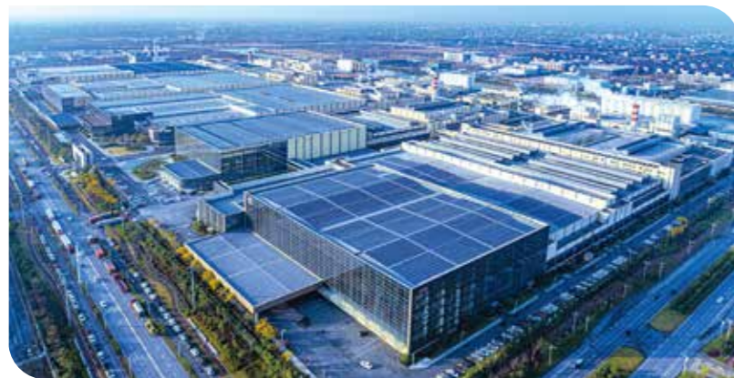
At the Tongxiang headquarters, the 600,000m 2 rooftops are fully outfitted with solar PV panels. These solar PV panels can produce close to 70 million kWh of energy per year, which is exclusively used for production.
