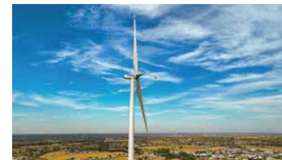
Hoisted wind turbine generators.
