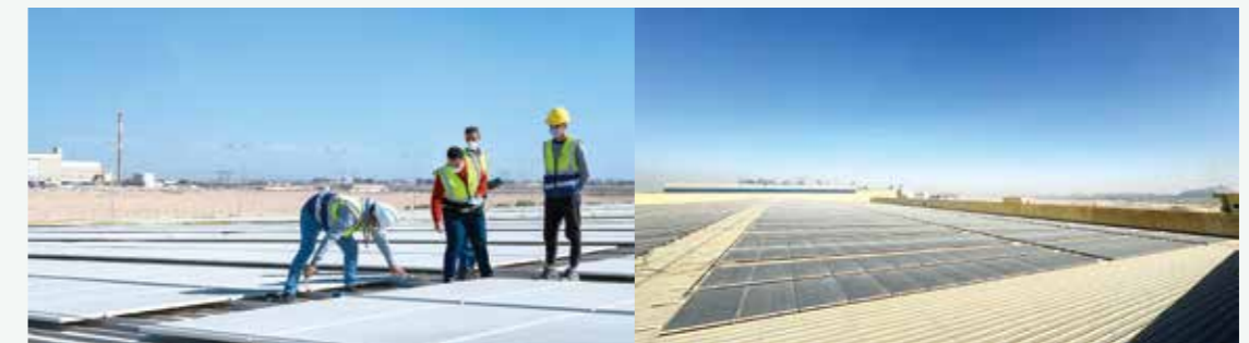
Jushi Egypt built a photovoltaic power generation project.
